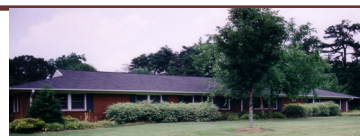
The Duke Street Supported Living Program provides housing for developmentally disabled.
